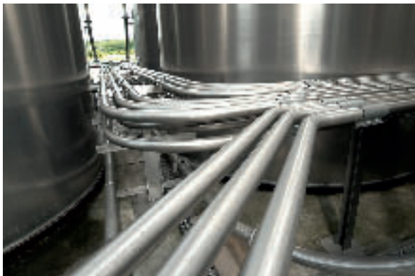
Customised routes of piping shaped on site
