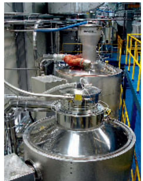
Receivers for flakes and granules on drying hoppers
