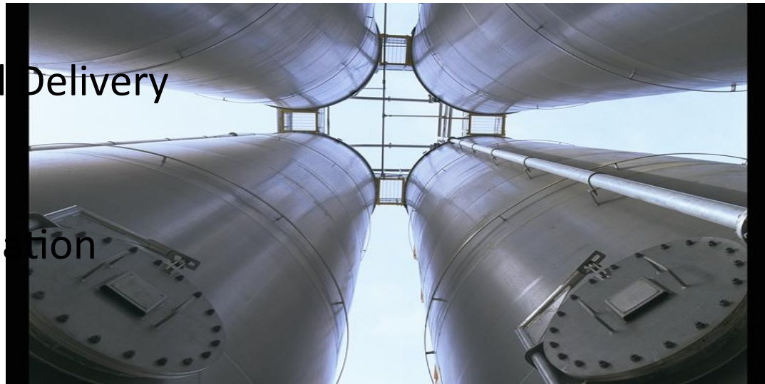
Shell Manways on 400te Silos
