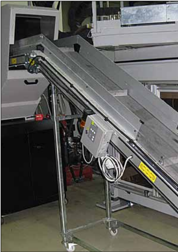
Machinery protection. Plate type metal detector ELCON installed on the conveyor belt leading to the granulator.
