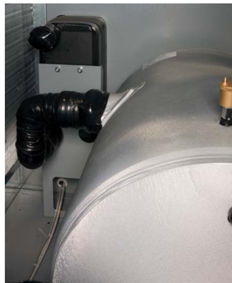
Insulated stainless steel brazed-plate evaporator
